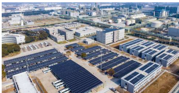
Covestro's Shanghai integrated site's large-scale distributed photovoltaic power facility has been recently commissioned, with an expected annual power generation of 6 million kilowatt-hours.
